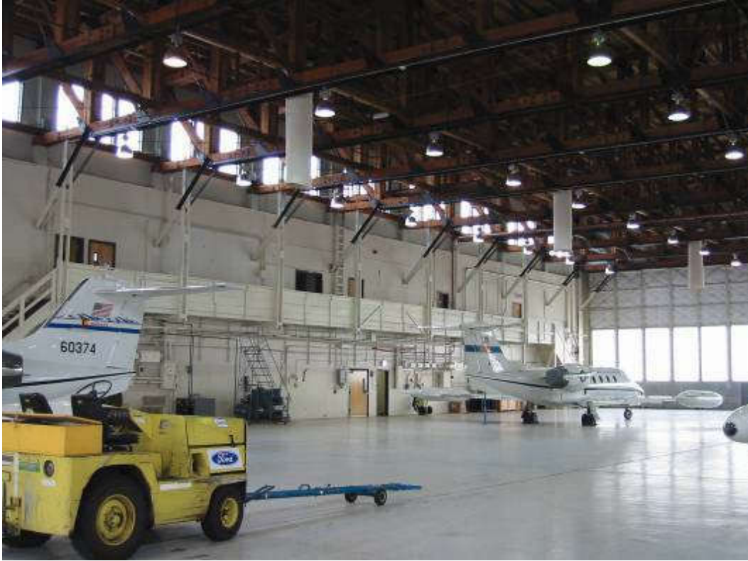
Figure 12 Example of Clerestory Application
